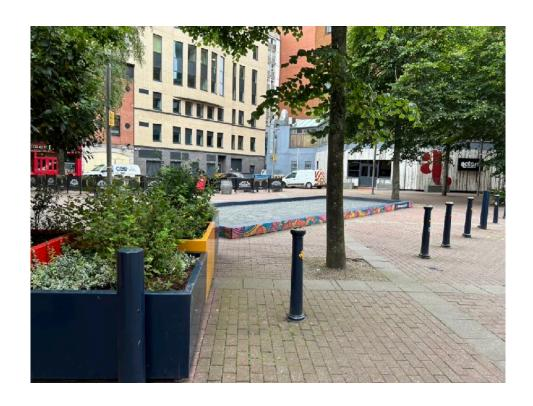
The junction of Amelia Street, Brunswick Street and Franklin Street is a raised table contiguous with the east boundary of the Square. Although tactile paving has been provided to indicate uncontrolled crossings the flush surface with the carriageway throughout this space makes finding the crossing points extremely challenging for people with a visual impairment and the junction design is dangerous and confusing for these users.
