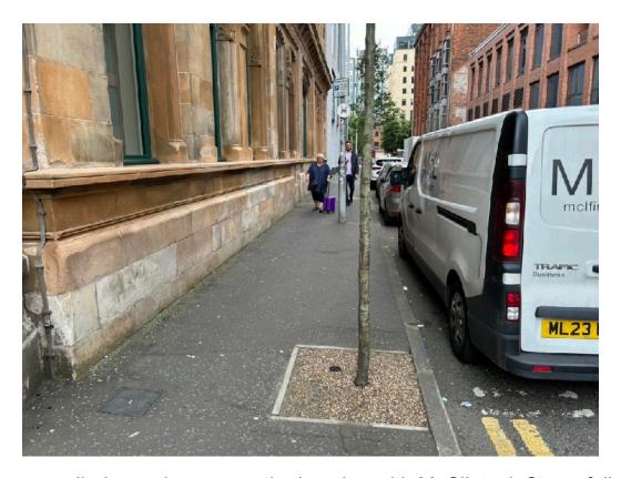
The uncontrolled crossing across the junction with McClintock Street fails to provide the required step free access. Damage to tactile paving indicates frequent mounting of the footway by heavy vehicles.
