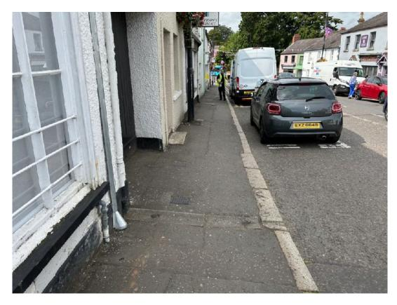
Footway conditions are poor in places along the southern footway and the use of dish drainage channels on both sides impacts on pedestrian comfort and accessibility.
