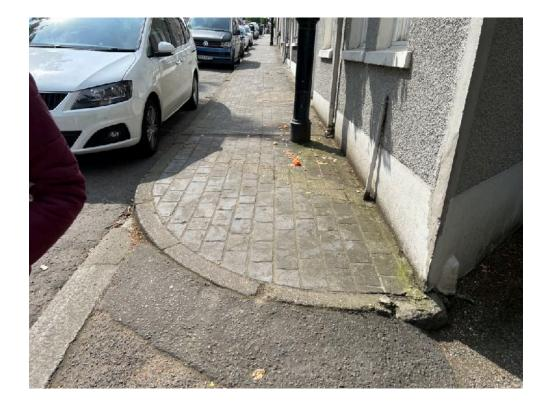
The wider condition of the footway is mostly satisfactory, although the use of dish drainage channels impacts on the comfort of the footway for some users.
