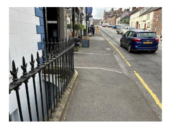
Footway condition is poor in places, particularly around vehicle entrances. Although for the most part step free access is facilitated, the steep gradient of the street has made provision less than ideal in places.
