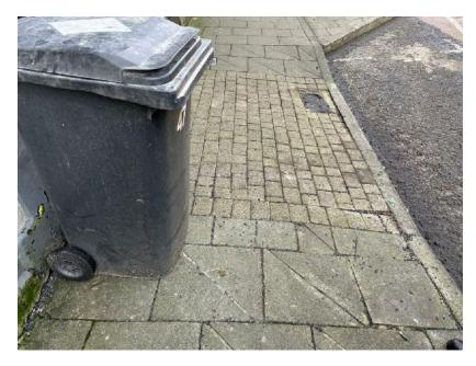
Image shows a sharp crossfall on the footway on Castle Street created by a dropped kerb at a vehicle entrance. The gradient of the street exacerbates the fall.
