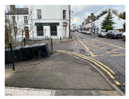
Image shows poor surfacing on the footway at a vehicle entrance at the junction of Ann Street and Station Road. No tactile paving has been provided on the northern footway for crossing of Station Road. Bins and railings narrow pedestrian accessibility on the junction crossing.
