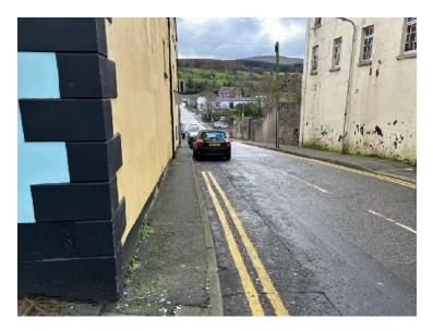
Image shows the narrow footway widths on Fairhill Street which provide a pedestrian route from the public car park. The footway also has a poor surface.
