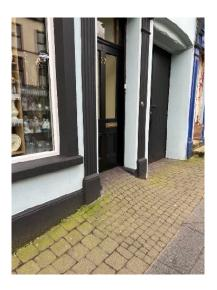
Image shows attempts to provide step free access to premises on Ann Street with a steep, short ramp (stepped access to adjacent buildings is just visible).
